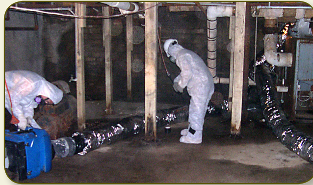
Workers remove mold and asbestos from the basement under the stage.
